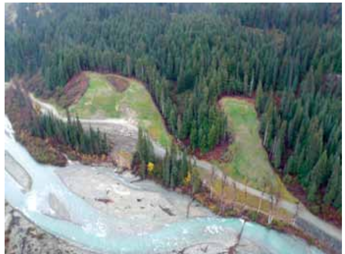
REVEGETATION PROGRESS ON CUT SLOPES ALONG THE GALORE CREEK ACCESS ROAD
